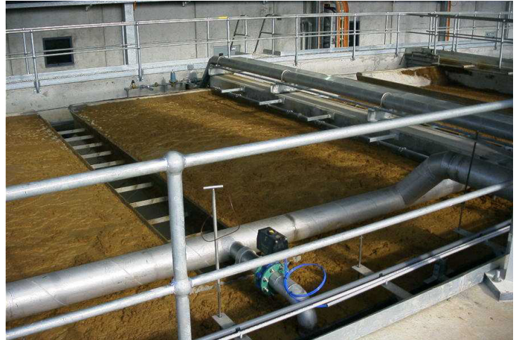
DAFF with hydraulic sludge decanting
